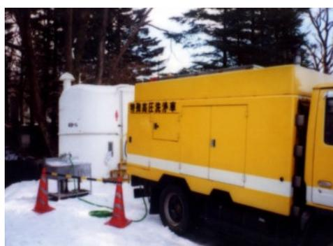
Figure 9 · 10 – Maintenance of re-circulating toilets at a ski area
